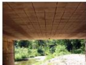
a) Grooves Prepared as per Design Geometry
