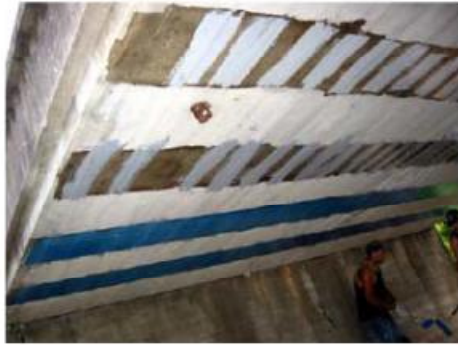
i) Surface Preparation with Primer and Putty
