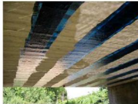
d) Application Completed
