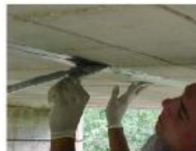
b) Inserting Epoxy Paste into the Groove
