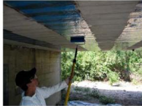
b) Application of Saturant
