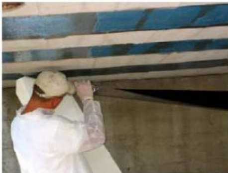
c) Application of CFRP Laminates
