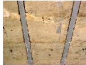
d) Application Completed
