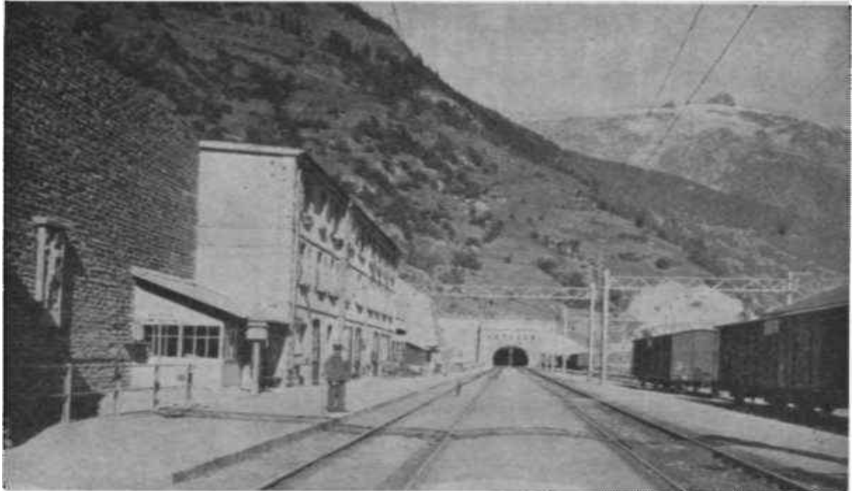
Goppenstein Station, southern entrance to Loetschberg Tunnel, Swiss Federal Railways.
