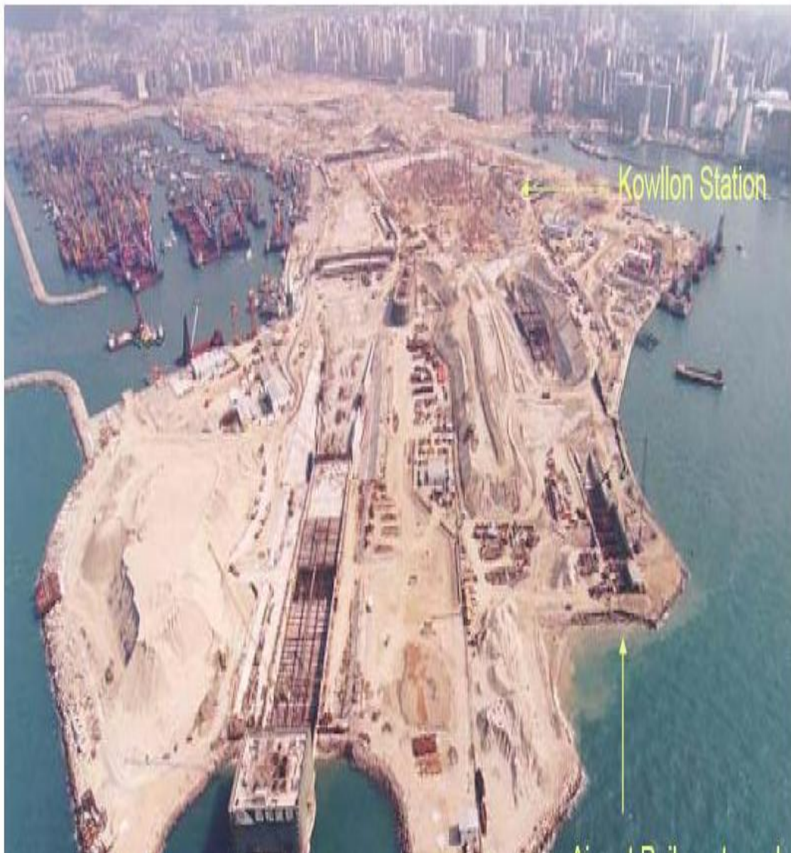
Airport Railway tunnel
