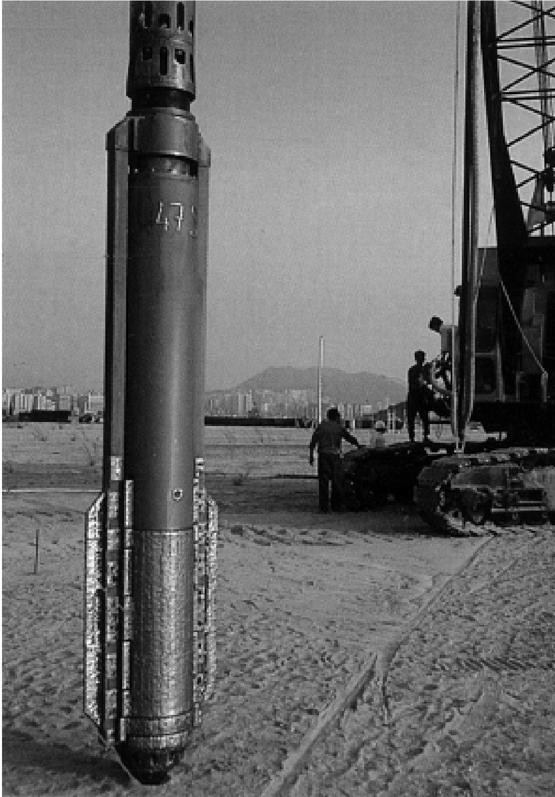
V23 at West Kowloon Reclamation
