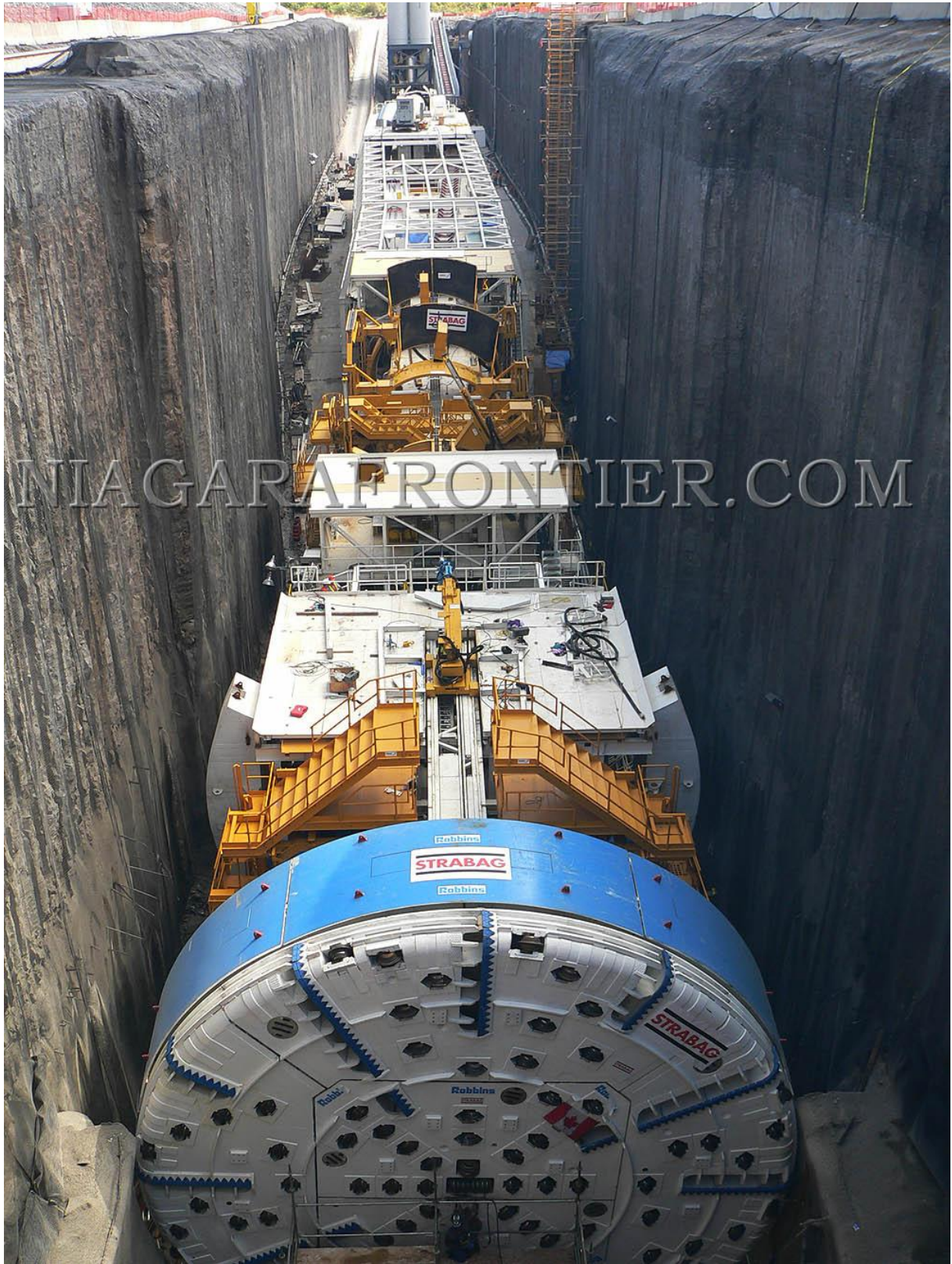
Tunnel Boring Machine
