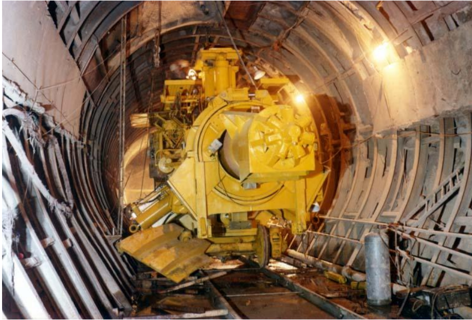
Tunnel Boring Machine
