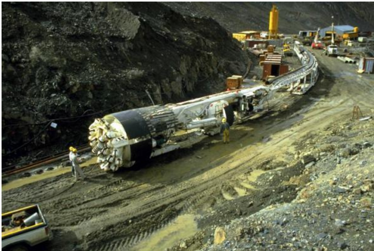
Tunnel Boring Machine
