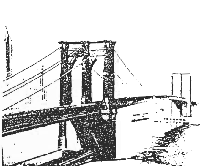
Σχ.1.14. Γέφυρα Brooklyn (1870-83)
