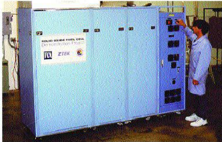
Testing of the 25kW power system.
