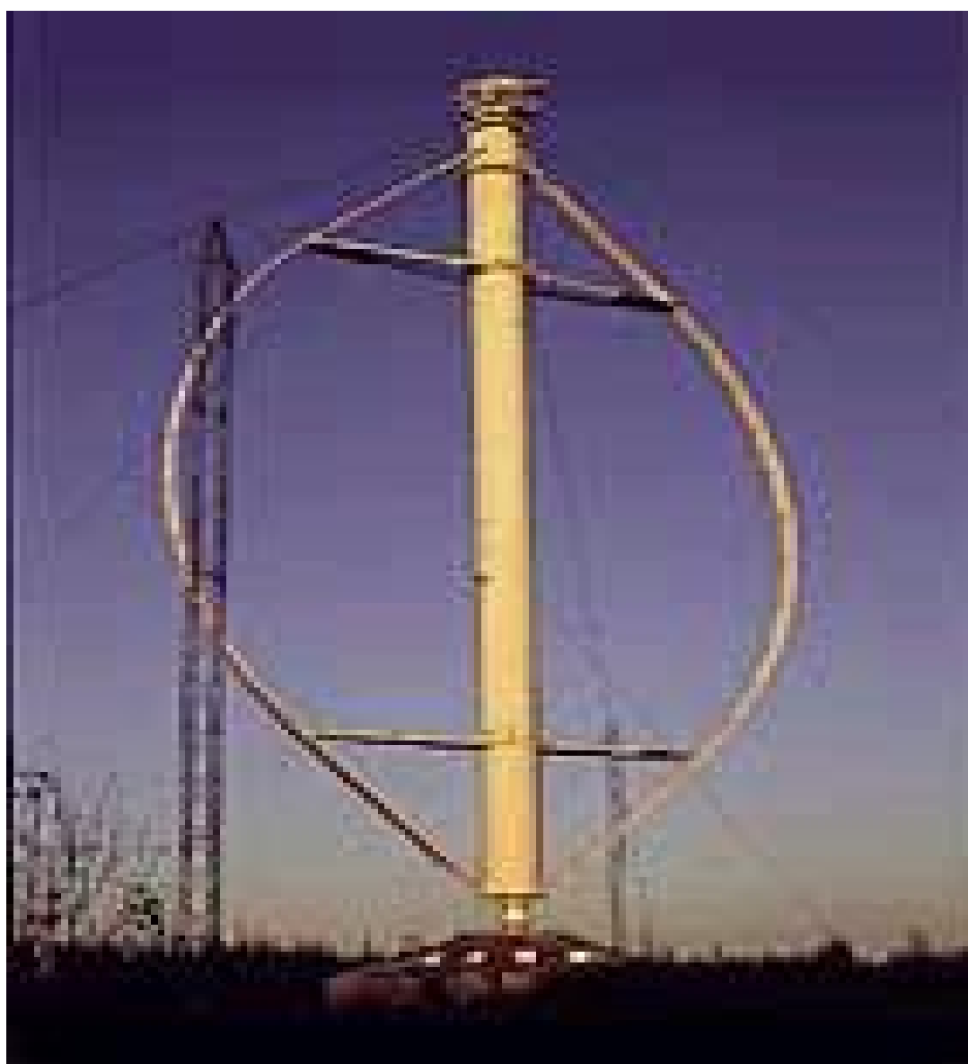
Figure 1-2. Eole C, a 4200 kW vertical axis Darrieus wind turbine with 100 m rotor diameter at Cap Chat, Québec, Canada. The machine, which is the world's largest wind turbine, is no longer operational. From www.windpower.org (2000), © Danish Wind Turbine Manufacturers Association.
