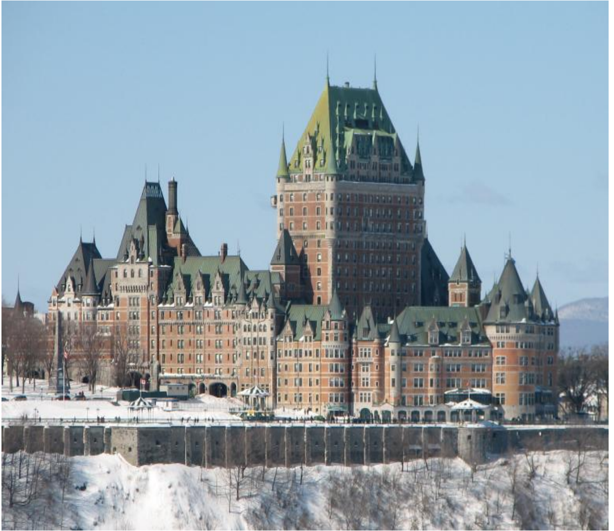
Fairmont Le Château Frontenac Quebec Hotel
